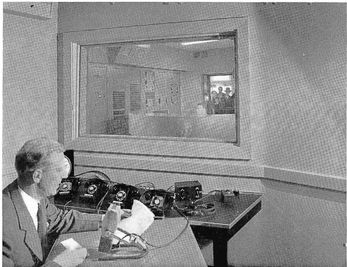
FIG. 44. Radio master control room at WCAU. Console is a deluxe RCA unit custom built for WCAU. Racks of RCA amplifiers and other units at the right form the wall between the control room and the equipment room which is located between the radio and TV master control rooms (see Fig. 46).
