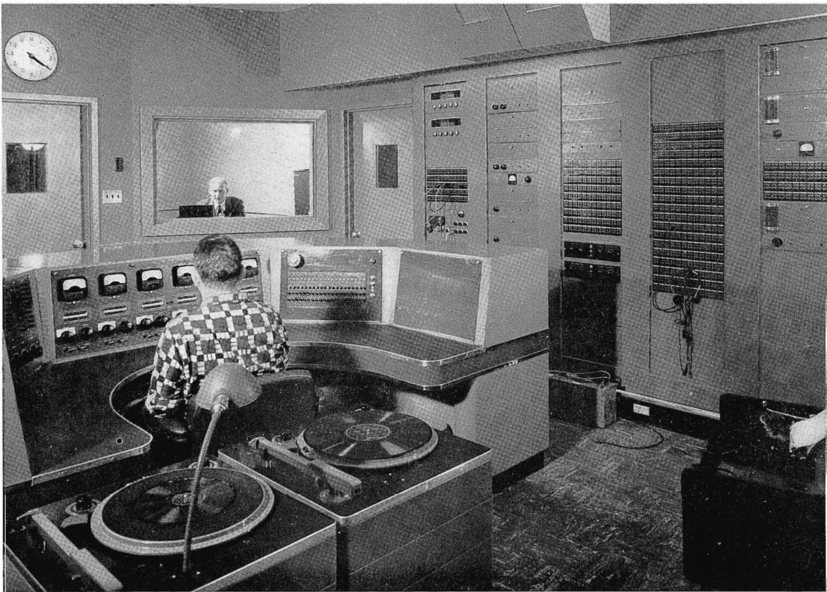
FIG. 44. Radio master control room at WCAU. Console is a deluxe RCA unit custom built for WCAU. Racks of RCA amplifiers and other units at the right form the wall between the control room and the equipment room which is located between the radio and TV master control rooms (see Fig. 46).
